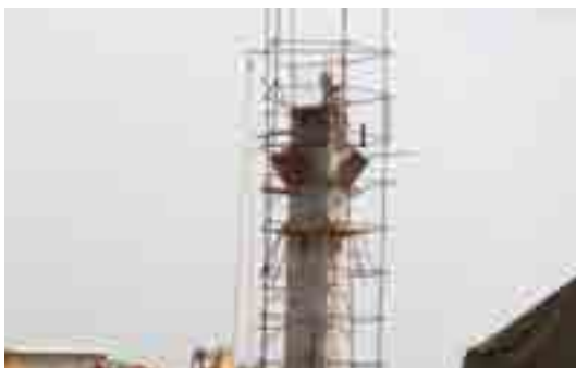
In 2017 we entered into an agreement with the Ivorian government to improve access to water around the Tongon mine.
