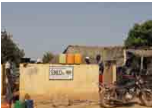
During 2017 we built or rehabilitated 70 boreholes for our local communities.
