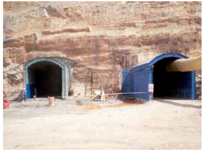
In preparation for the Gara underground mine at the Loulo complex, the decline development has increased and both portal frames (shown) have been put in place to secure the entrances.
