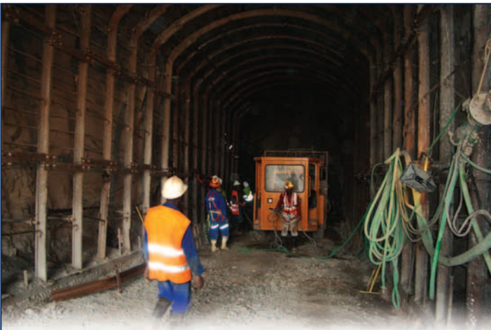
Yalea underground development: installation of supports for decline.
