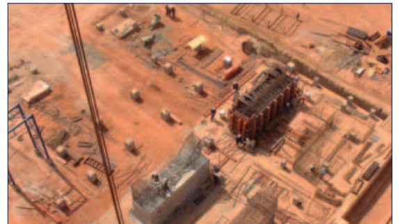
Building a mine - Loulo 2004.
